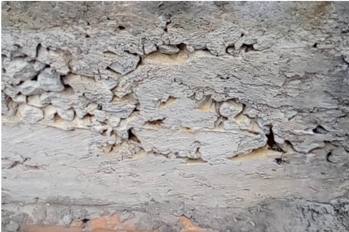
Photo plate 10: Honey combings observed in some area.
