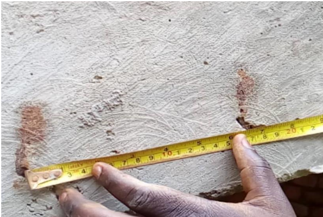
Photo plate 07: Reinforcement bar details being captured
