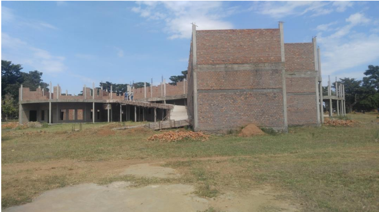
Photo plate 01: the as built structure under investigation.
